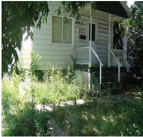
Pictured above is an abandoned home with an overgrown lawn.
